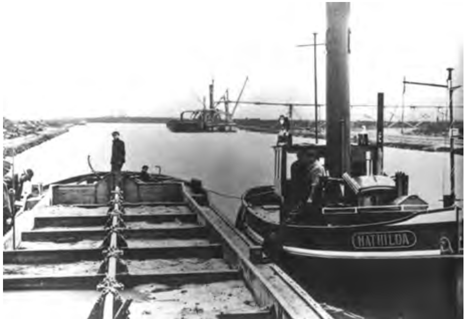
MATHILDA was the first tug owned by Antonie Kooren and is seen here alongside a dump barge. On the left the height of the sand in the hold is measured to determine the total load and thus the value of the 'cargo'. In the distance a barge-discharge dredger is waiting to pump the sand ashore photo: coll. Job van Eijk
