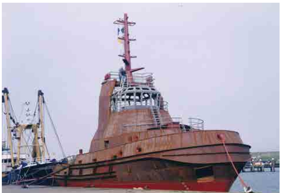
RT MAGIC under construction at the Padmos yard
