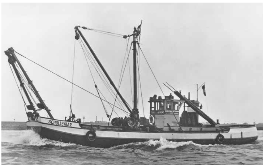
Like ZEELEEUW, SCHOLLEVAAR was also employed in the 1940 wreck removal / gold salvage operation. Built 1940 - 60 bhp - 20,01 x 5,50 m. 1943 NT 45 for Kriegsmarine. 1944 BS 41 (Bergungsschiff Verband). 1945 aagain Taksberging. 1969 sold for scrap photo: postcard issued by W.A. van den Tak
