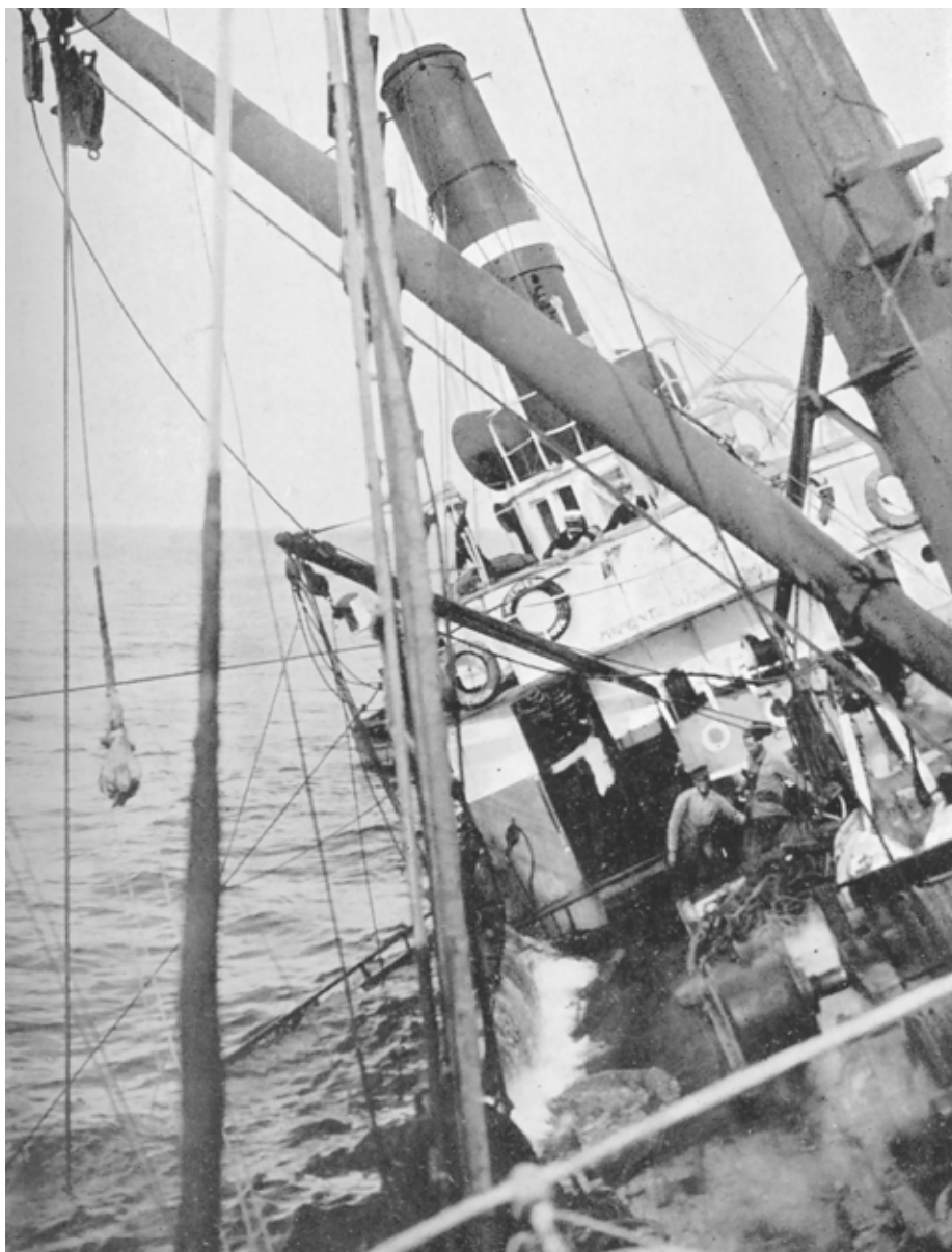
ARTIGLIO at work tearing material from the hull of a wreck
