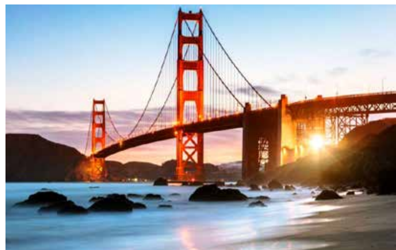
Golden Gate Bridge
