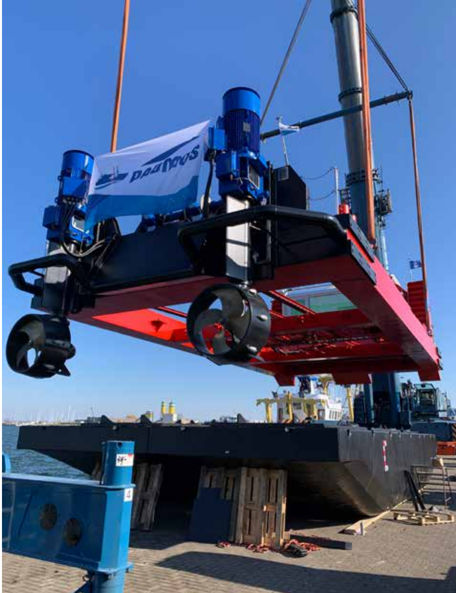
The hull frame about to be lowered on the hull cubes. Propeller pods already bolted on photo: Kotug / Bas van Hoorn
