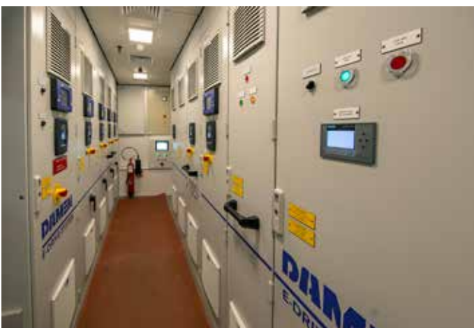
Switchboard room on board SPARKY
