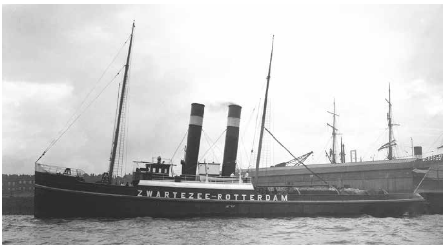
ZWARTE ZEE was completed in 1906 by J.& K. Smit, Kinderdijk for account of L. Smit & Co. 51,70 / 50.14 x 9,15 x 5,29 m. Draught 4,60 m. 1.250 ihp. 1914-1918 Royal Dutch Navy as inspection vessel. 1933 sold to Bugsier as ALBATROSS. Reconstructed with single funnel. 1939-1944 Kriegsmarine. Twice sunk and raised. 1945 French Government, renamed TAUREAU. 1946 scrapped. Photo dates from WW-1 - see neutrality markings
